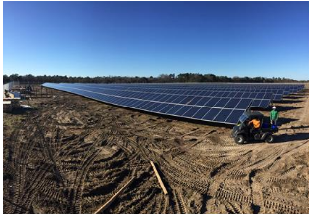
EXAMPLE OF A SOLAR PROJECT IN CONSTRUCTION
